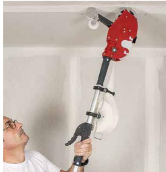
To apply tape to the ceiling, install the extension of your choice depending on the height and access. Possibility of working at heights of 3 metres.
