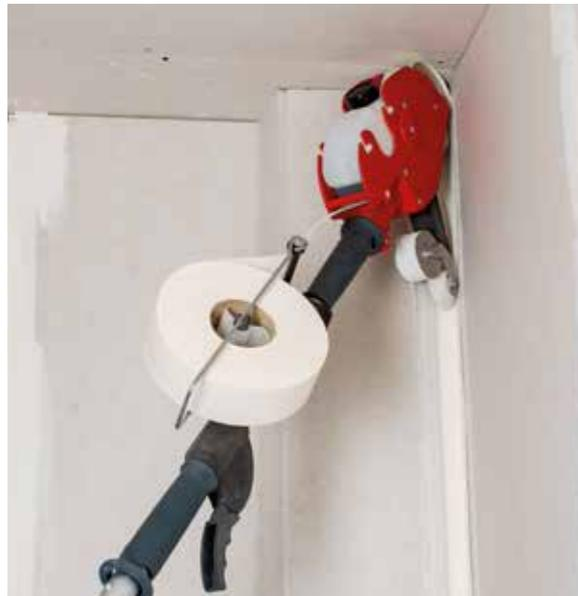
When applying the corner tape from bottom to top, swap the rollers. The tape is automatically shaped to fit the angle. Top tip: the corner DécoLiss® is designed to smooth out the tape and facilitate wiping down.
